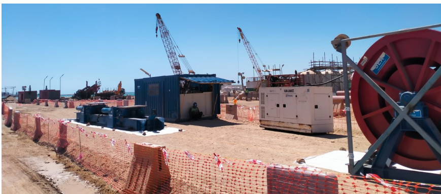
Pulling Spread at Worksite
