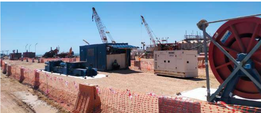
Pulling Spread at Worksite
