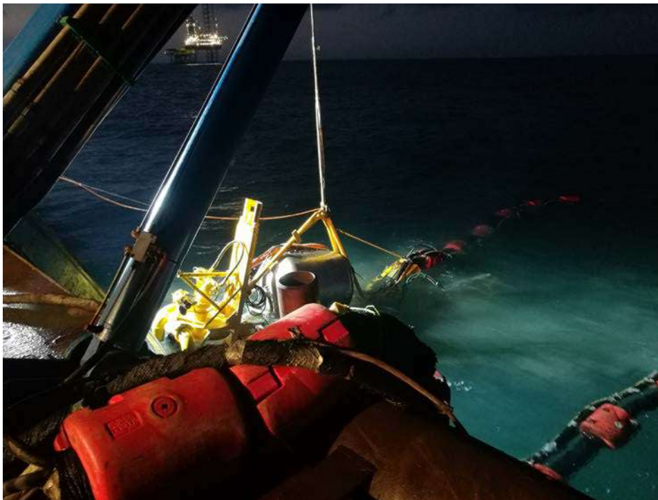
LEO PTM during XANAB trenching operations - by night.
