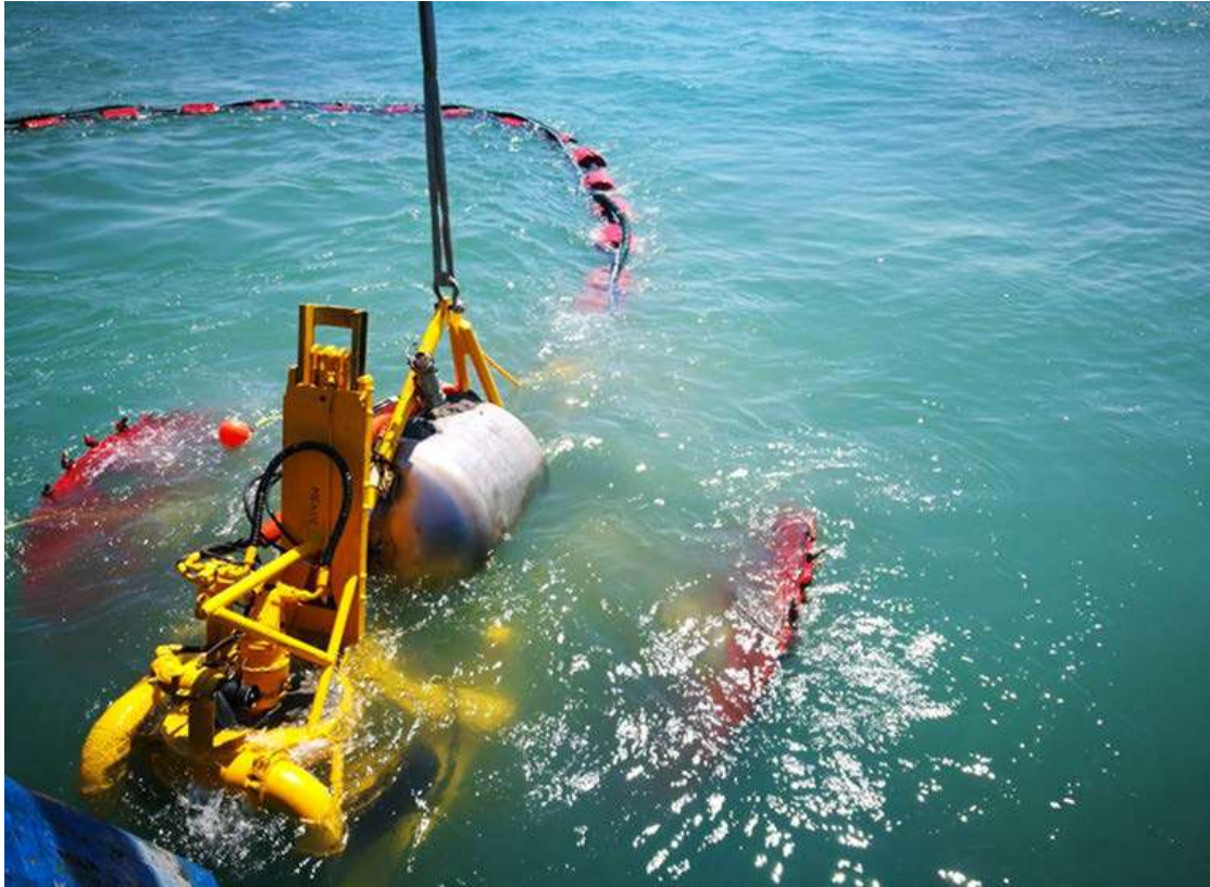
PTM in the water during trenching operations
