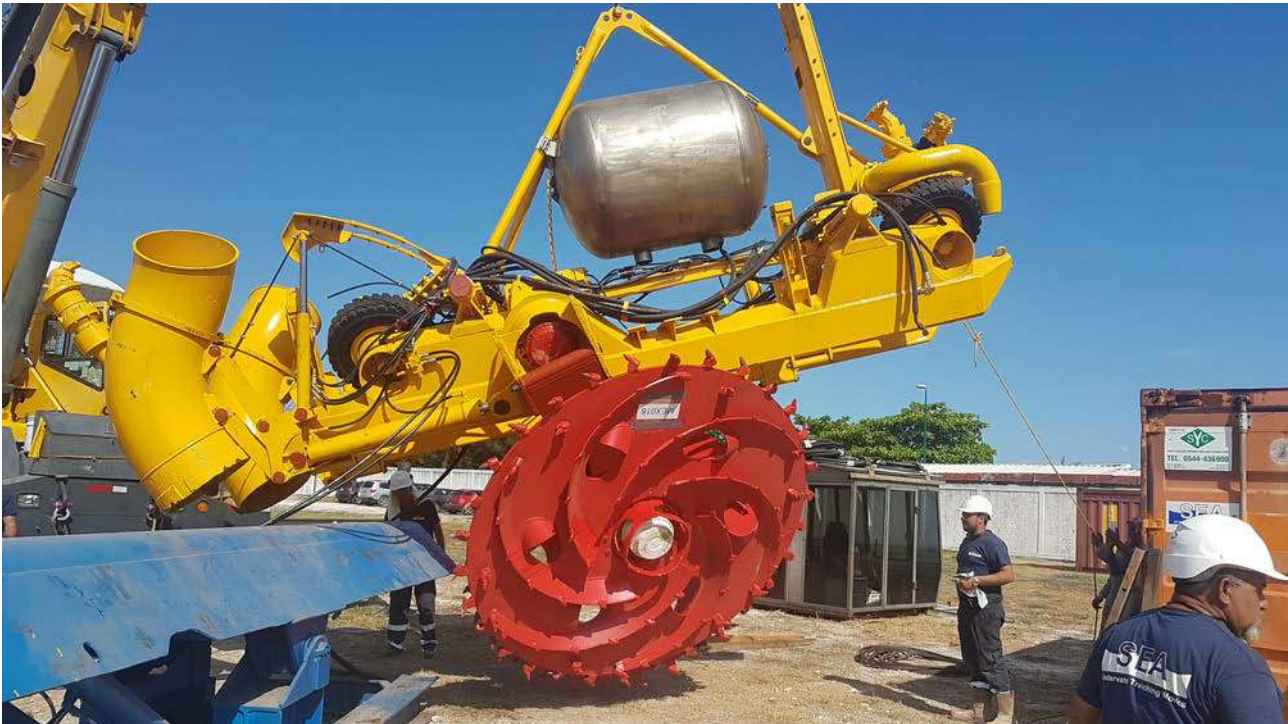
PTM during assembly phase onshore
