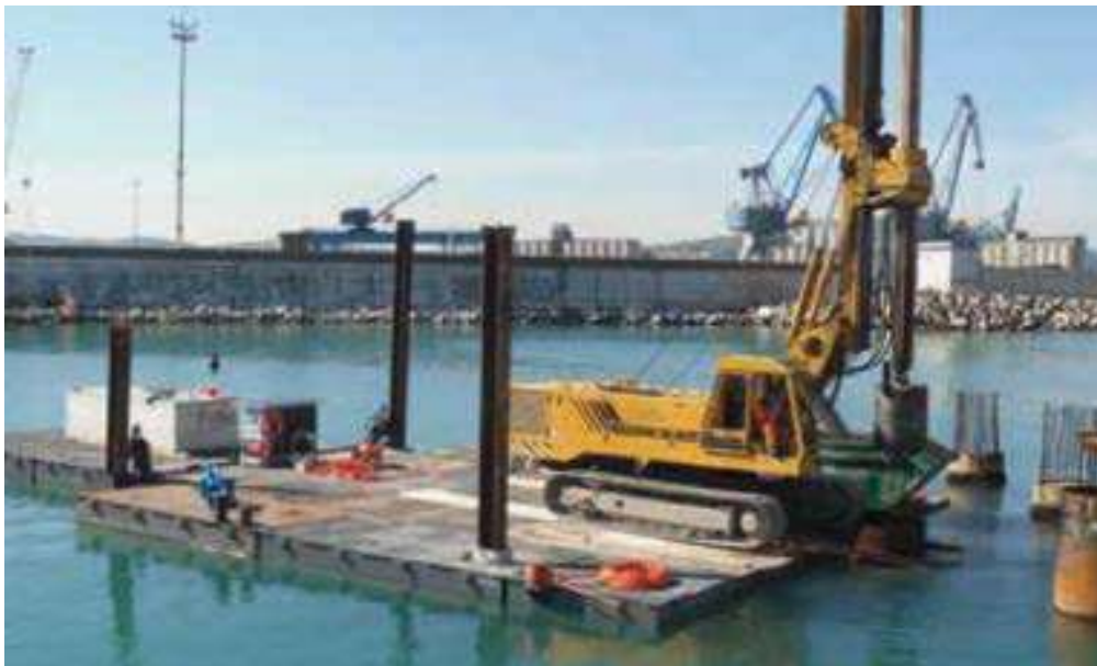
The modular pontoon for shore approach
